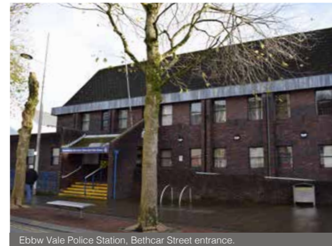
Ebbw Vale Police Station, Bethcar Street entrance.
