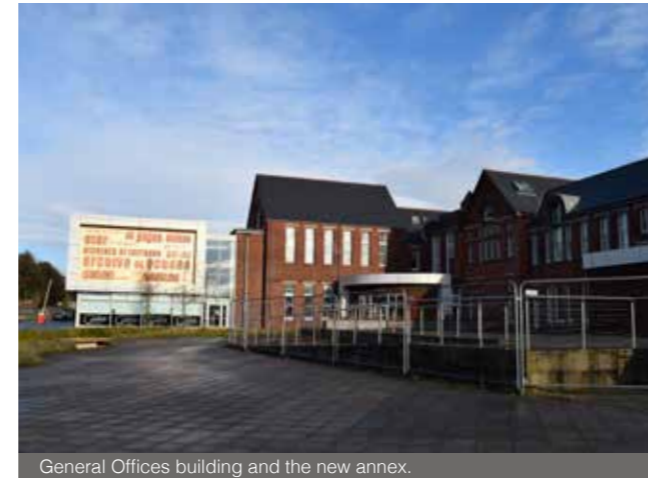
General Offices building and the new annex.
