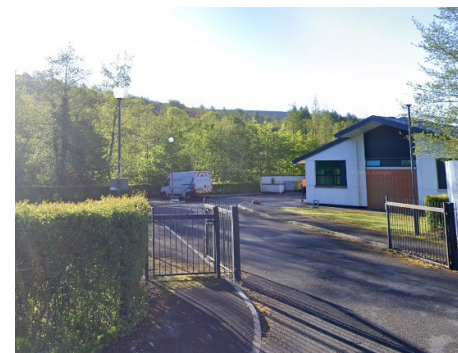
Augusta House, Ebbw Vale
